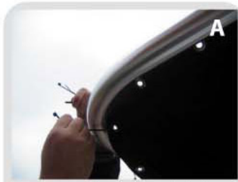
Temporarily fasten fabric to frame by wire tie or rope.
